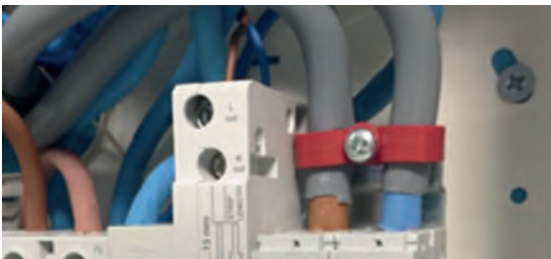
Fig 16. Example internal meter tail clamp
